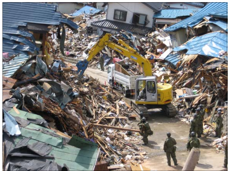
The process was carried out very carefully, for there were still family members missing under the rubble
